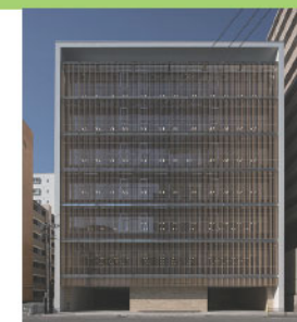
Higashi Hie Business Center III
