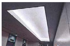
Example of shifting to LED lighting at Sanix Hakata Building
