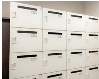
Installation of personal lockers
