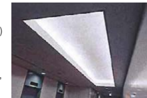
Example of shifting to LED lighting at Sanix Hakata Building
