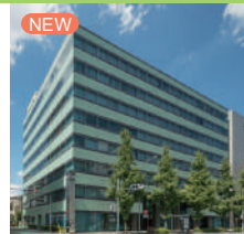
NEW Hakata Chikushi-Dori Center Building
