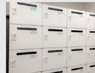
Installation of personal lockers
